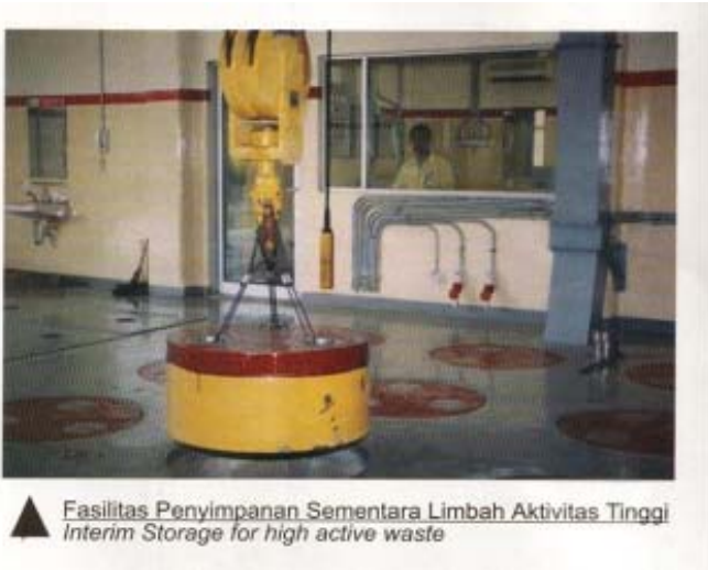
Fig. 3. Interim Storage for High Active Waste (Capacity 120 drums)
