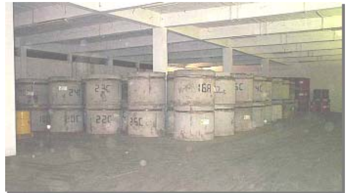
Fig. 2. Interim Storage Building No. 1 with total area 1420 m 2 and capacity 420 drums, 90 concrete shell
